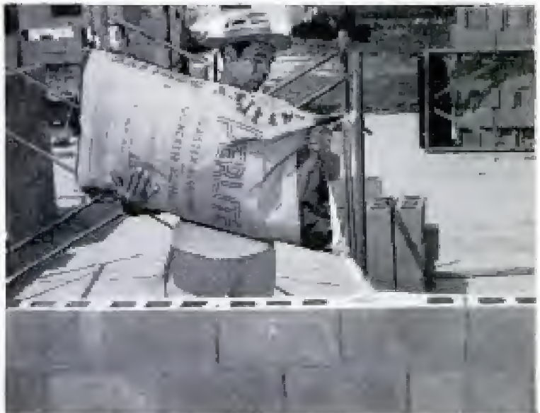
Perlite core fill for concrete blocks can double insulating effect of wall. Perlite insulation can't rot, decay or settle. Spraying machine below does the work of four plasterers. Light weight of plaster made with perlite makes spraying possible
